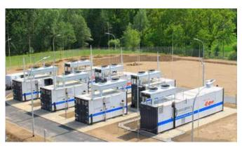
**Figure 9:** 2MW Power to gas unit based on alkaline electrolysis in Falkenhagen, Germany. The hydrogen is injected into the gas grid without methanation. (Source: E.ON)
