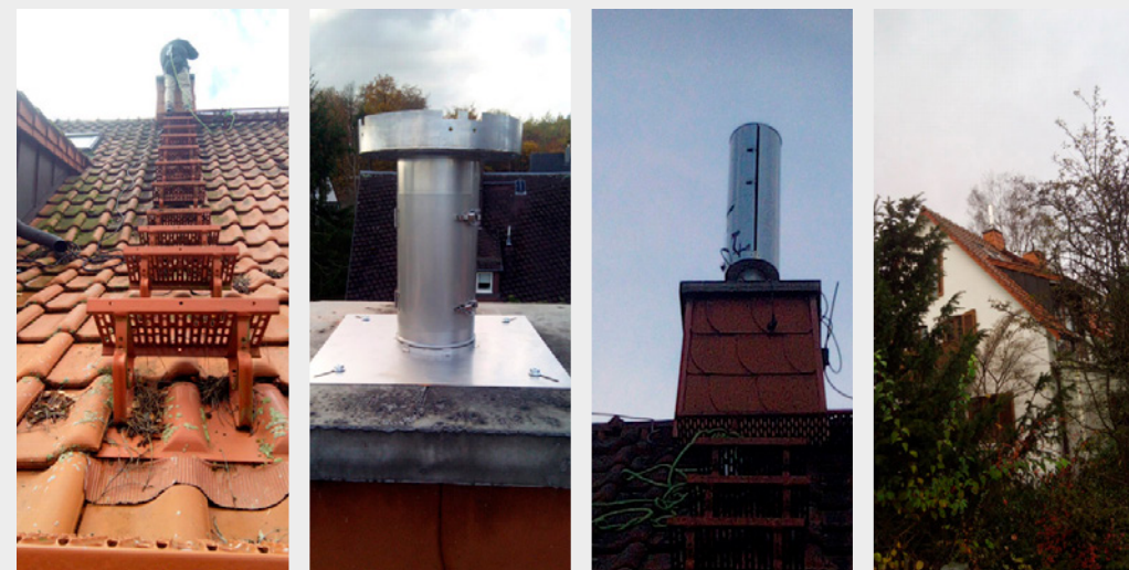
Fig. 25: ESP installation at a field site
