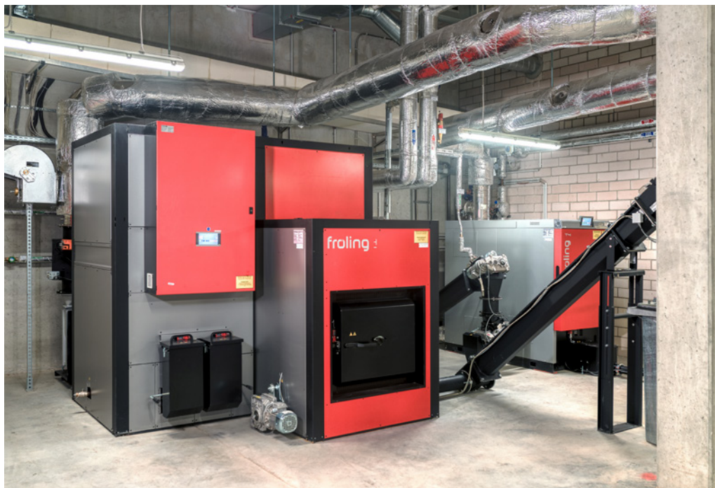
Fig. 14: Woodchip firing in the DBFZ technical centre
