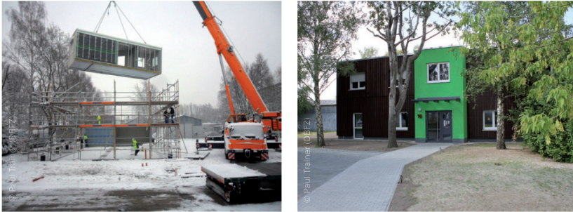
Figure 11: Construction of a new day nursery at the DBFZ facility
