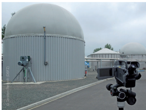
Figure 39: Use of an infrared camera to detect diffuse gas methane losses on the DBFZ biogas pilot plant
