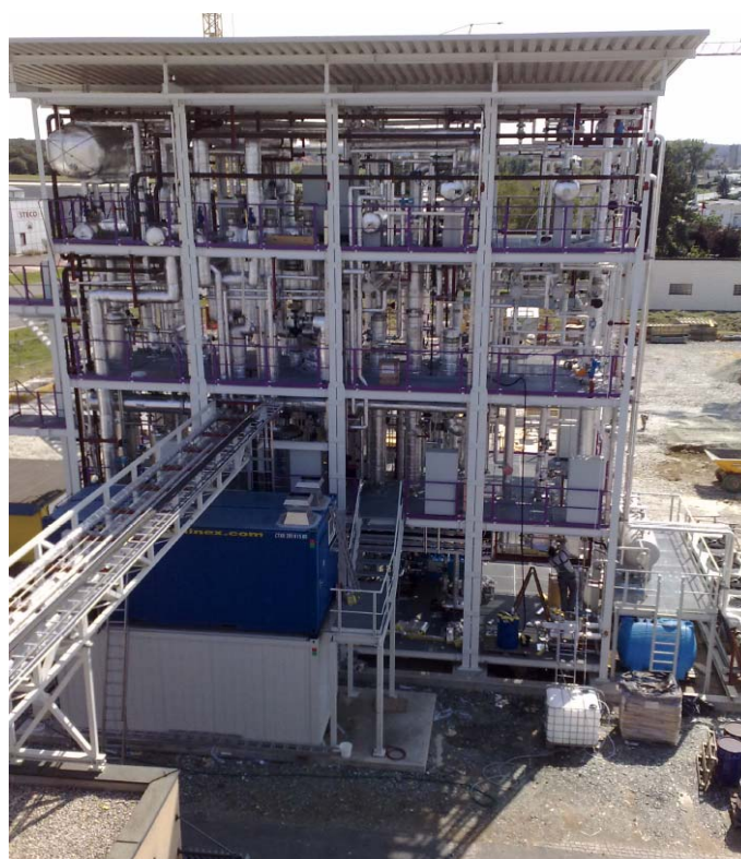
Figure 7: Completion of erection (2008-24-7)
