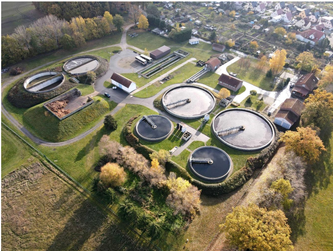
The Gröditz Wastewater Treatment Plant as an associate partner in the "ReKlär" project. Picture: © Heiko Brabetz
