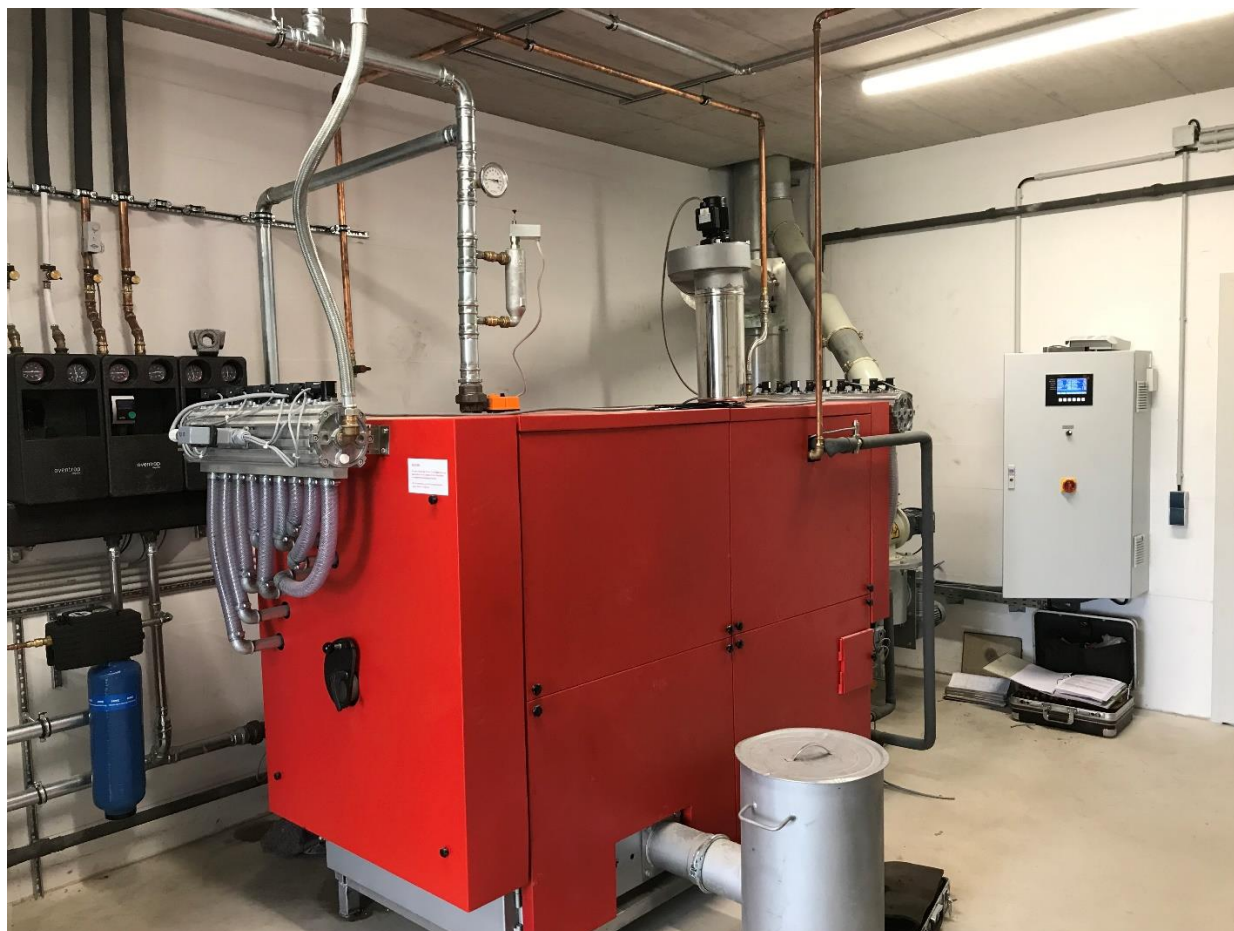
ÖKOTHERM® biomass boiler C1L (Source: A.P. Bioenergietechnik GmbH)
