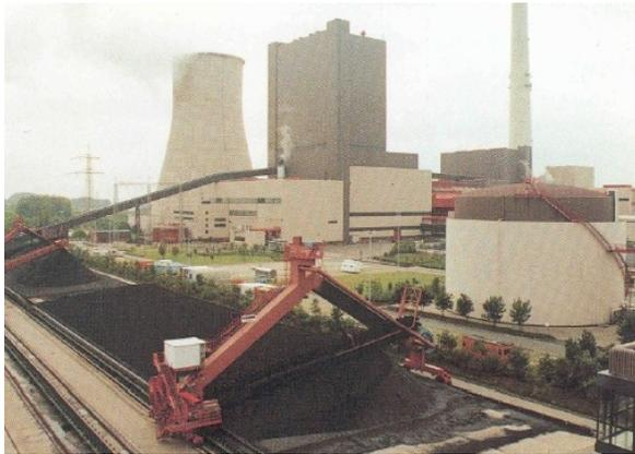
Figure 15: Outside storage with portal scrapers
