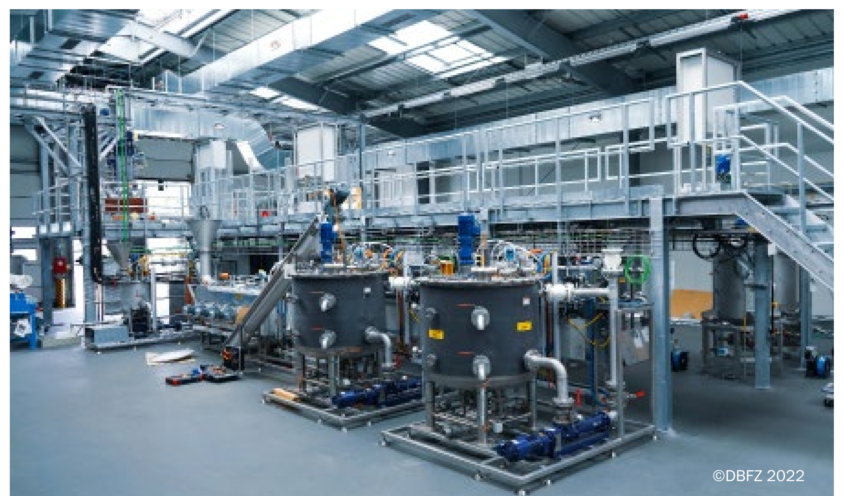
Fig. 3: Construction progress (anaerobic digestion line 2 with a plug flow reactor in the center of the photography)
