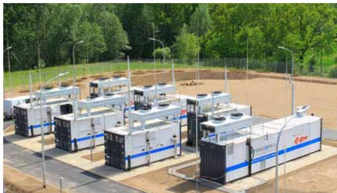
**Figure 9:** 2MW Power to gas unit based on alkaline electrolysis in Falkenhagen, Germany. The hydrogen is injected into the gas grid without methanation. (Source: E.ON)
