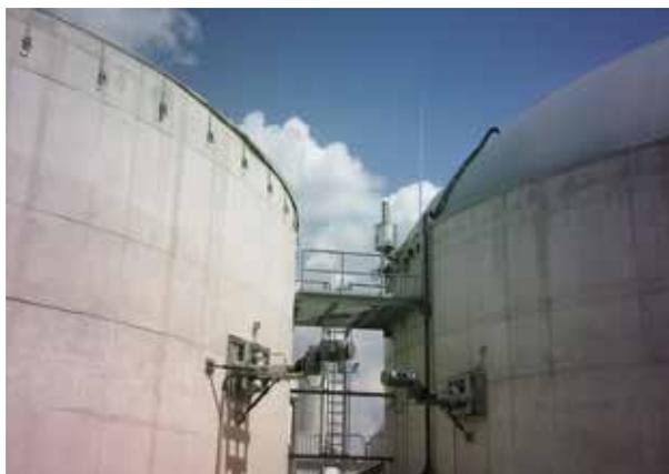
Figure 2: a) Point source pressure relief valve (PRV) (DBFZ)
