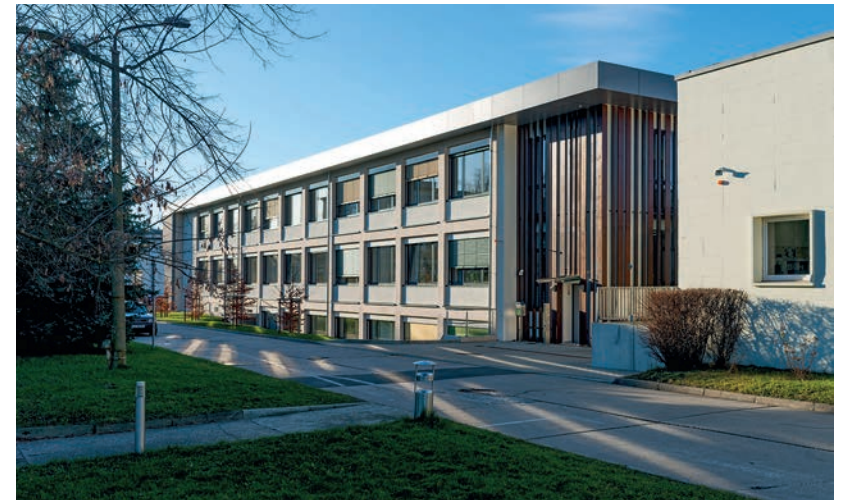
Fig. 42 The DBFZ main building in January 2015
