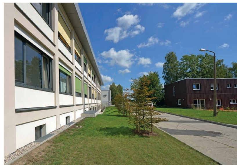
Fig. 50 The renovated main building of the DBFZ in Summer 2014
